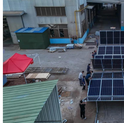
Pure Sinewave Inverter with Transfer Switch
