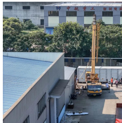
SUNWAY 30KW 51.2KWH Energy Storage System
