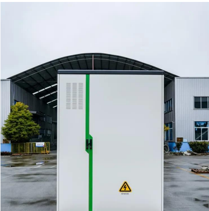
Solar PV Energy storage box installation and...
