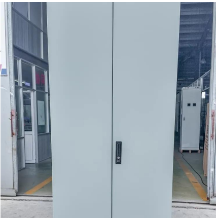
Containerized Photovoltaic Power Plant ...
