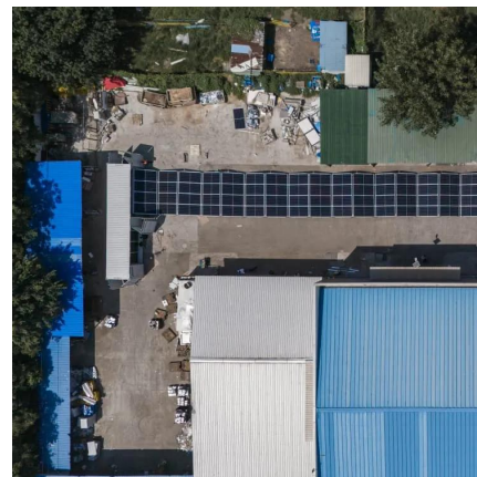
Al Hassan Switchgear Manufacturing Buyers: 6 Verified ...
