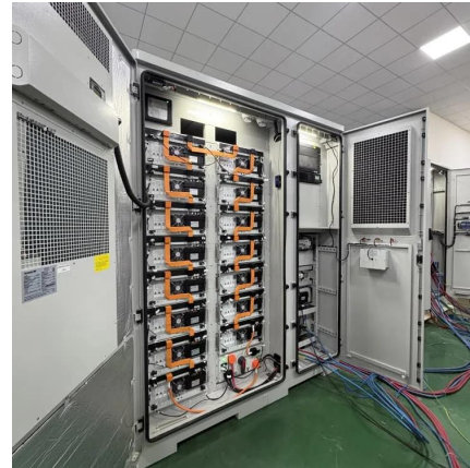
3kw off Grid Solar Power System
