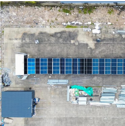
ASUNCION OUTDOOR ENERGY STORAGE CABINET QUOTATION
