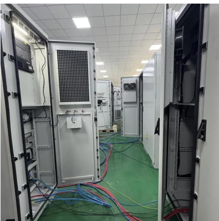
BLOEMFONTEIN LARGE MOBILE ENERGY STORAGE VEHICLE
