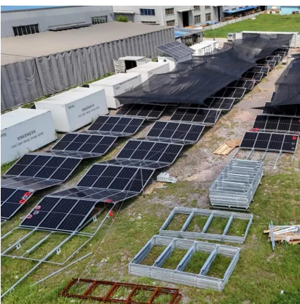
Protecting Solar BESS: Shipping Container ...
