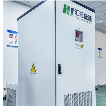
Bulwer Station Battery Energy Storage System ...
