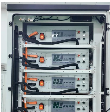
Solar DC Breaker - Zayel Solar
