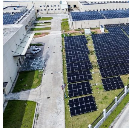
China Container Energy Storage System ...
