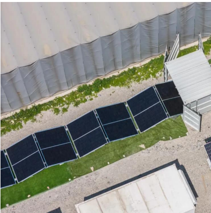
CAPE VERDE ENERGY STORAGE CONTAINER...
