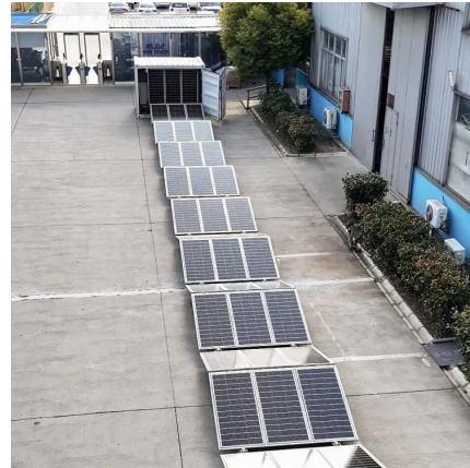
Ireland: top battery storage systems ...
