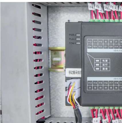
containerized battery storage , SUNTON...
