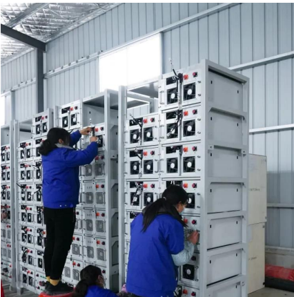
Solar Container , Large Mobile Solar Power ...
