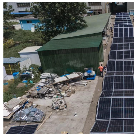
Latvia's largest battery energy storage system unveiled
