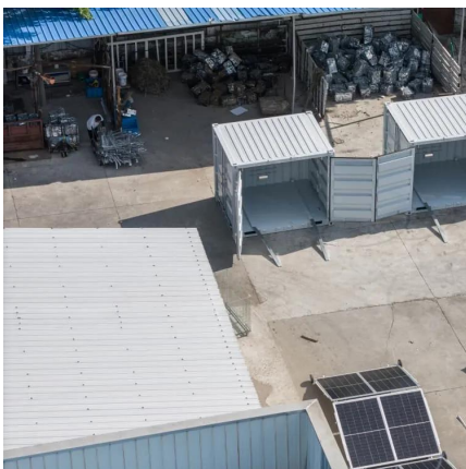
5G telecommunication base station solar ...
