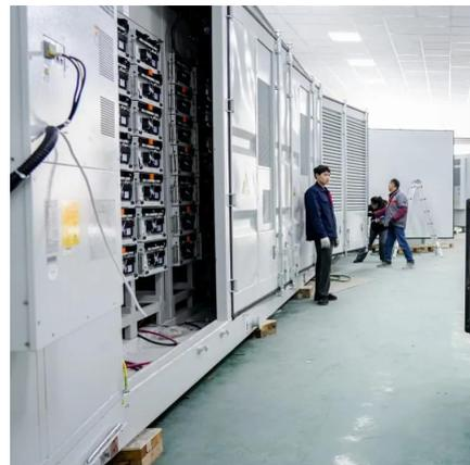
**200KWH commercial energy storage system\_Lithium Battery Storage Solar**
