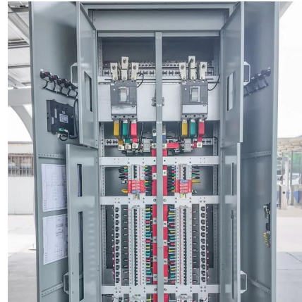
C& I ESS in Gothenburg office, Sweden
