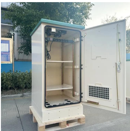
Dominican Republic advances in energy storage at Reform ...
