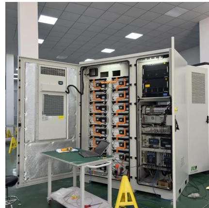
25kW Solar Wind Hybrid System for Remote Broadcast Station ...
