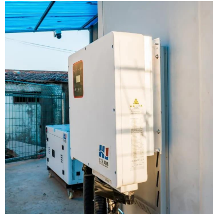
South Tarawa Full Battery Production Plant
