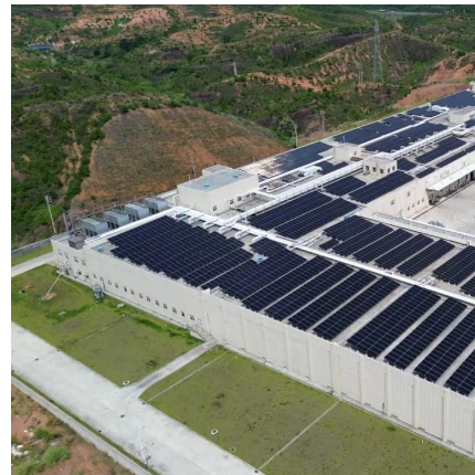
China's Largest Grid-Forming Energy Storage Station ...
