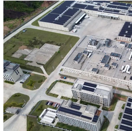
Vaduz Energy Storage Battery Solutions: Powering a ...
