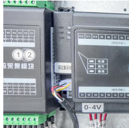
Zambia s first smart energy storage device
